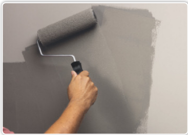
Step 4 - When the wall is dry, apply a second coat with a roller (PE15)
