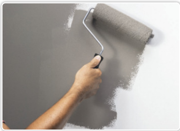
Step 3 - Apply the firsts coat with a roller (PE15), coverage 8/10 m²/lit each coat
